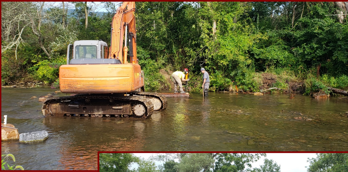
Yellow Creek work photos by Dave Wright.
